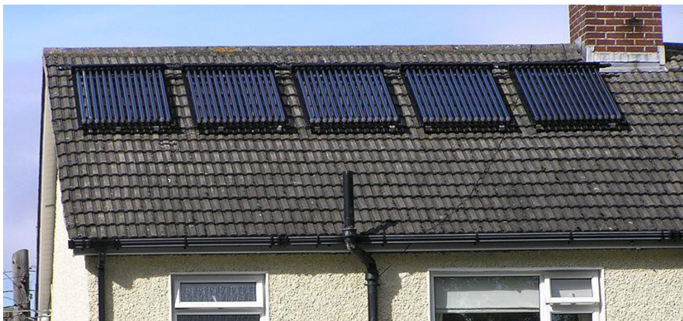
Figure 5 Domestic solar hot water panels (Copyright Terence Wiki and licensed for reuse under Creative Commons Licence )
