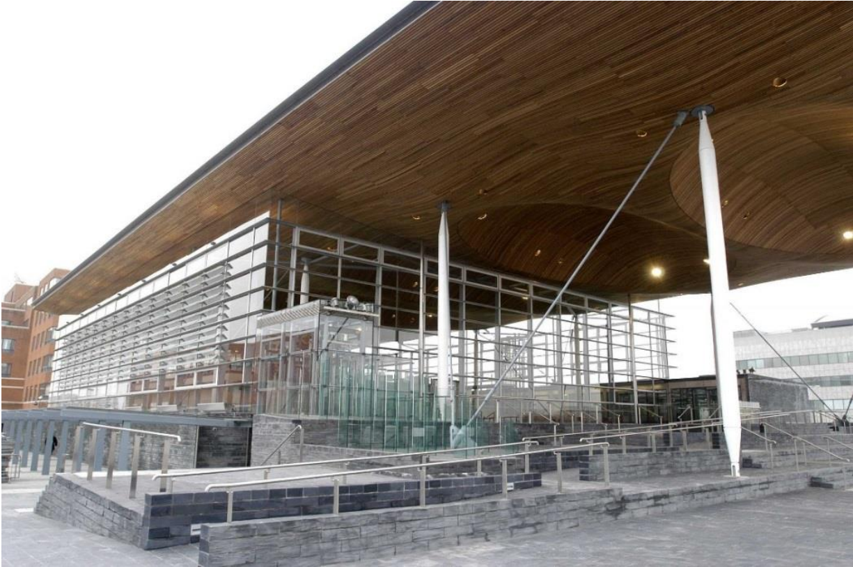
Figure 6 Senedd building made extensive use of wood as a building material and is heated entirely using a biomass boiler (Source: National Assembly for Wales)
