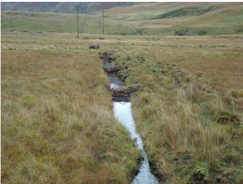
Ditches blocked on Dyffryn Mymyr to raise water levels and reduce erosion © NT
